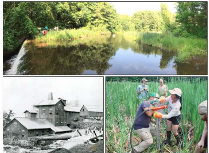
Figure 4. Top: Dam and sediment filled reservoir at the Buena Vista/Hunts Lyman Iron Company Furnace site on the Hollenbeck River in Canaan, Connecticut. Bottom: (left) Historical photo of the iron furnace, c. 1870 (courtesy of David M. Hunt Library) - note bridge over dam site in the foreground; (right) Keck Connecticut students vibracoring the reservoir sediment behind the dam in July 2015
