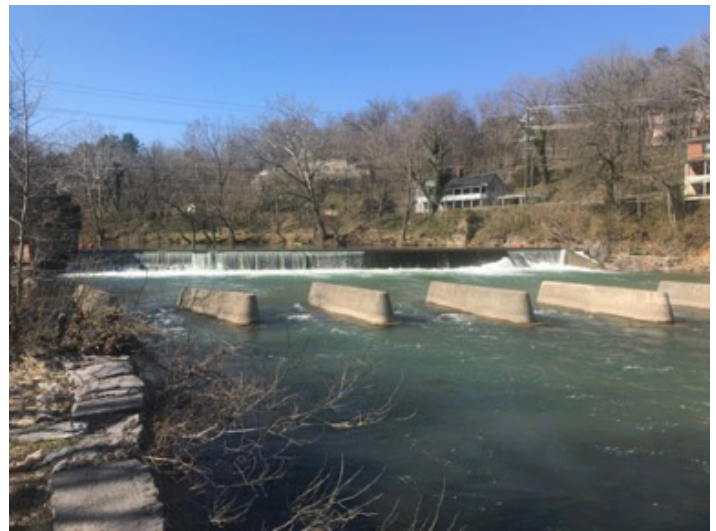
Figure 1. The Jordan's Point Dam, seen looking upstream, in March 2019. The structures downstream of the dam are concrete pylons, which were part of an old railroad bridge (Young, 2019); they have since been moved and now reside on river left downstream of the dam.
