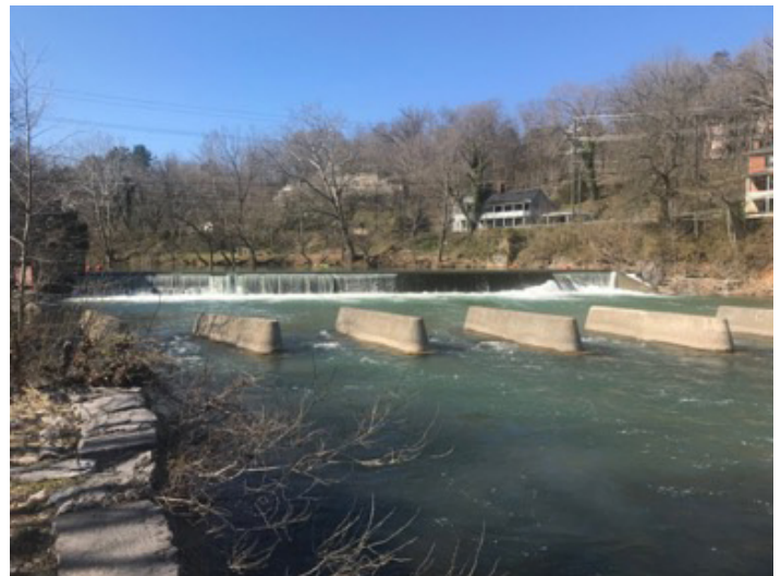
Figure 1. The Jordan's Point Dam, seen looking upstream, in March 2019. The structures downstream of the dam are concrete pylons, which were part of an old railroad bridge (Young, 2019); they have since been moved and now reside on river left downstream of the dam.
